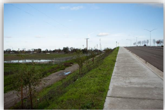
Figure 3 - Capital improvement projects such as roadways must include post-construction design measures and be appropriately sized.
